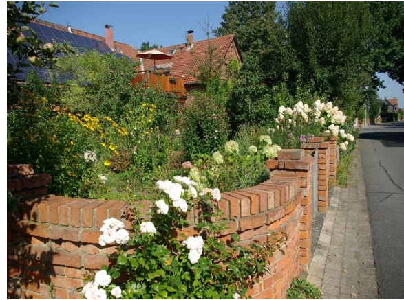
Abb. 4-16 Ziegelmauer in Immensen
